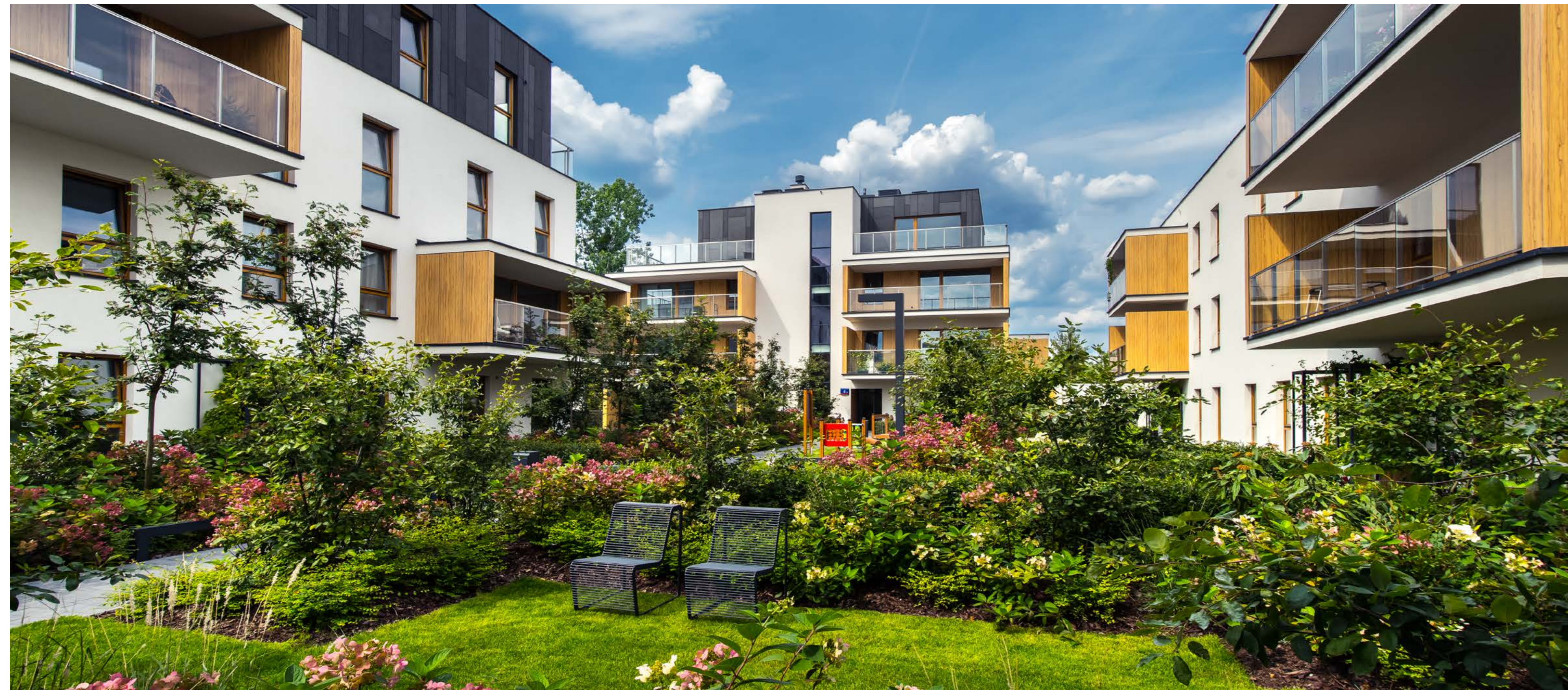
APARTAMENTY MARYMONT by Matexi in Warsaw, Poland
